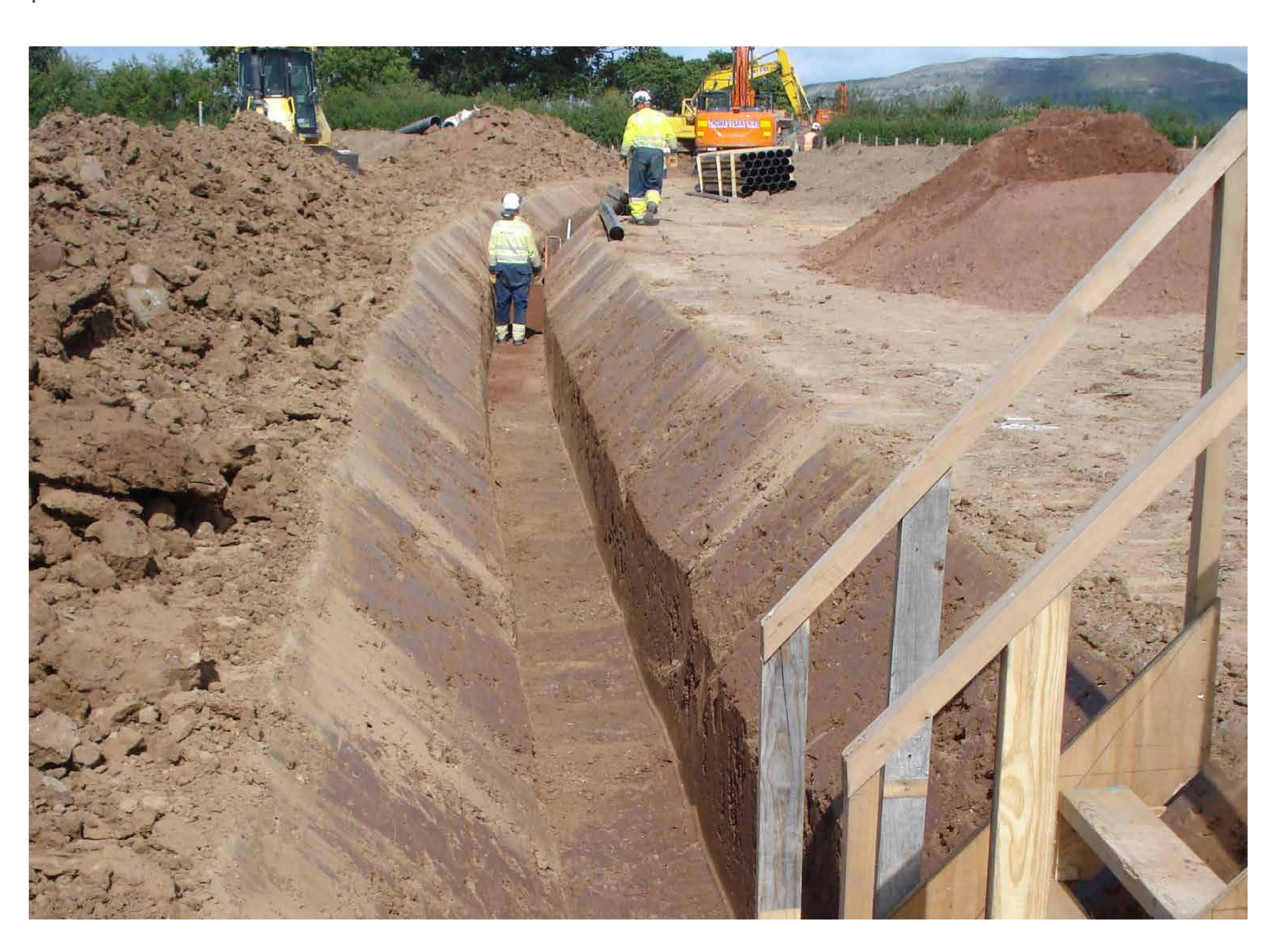
At certain locations, alternatively bespoke tools may be used. These are usually tracked vehicles, that excavate a trench, lay the cable, and then bury the cable simultaneously. Alternatively, they may excavate a trench in advance, then lay the cable after it is pulled into the Transition Joint Bay (e.g. at the landfall).
